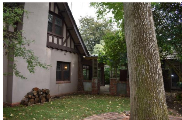
View of rear extension and verandah (source: Extent Heritage Pty Ltd, 2022).
